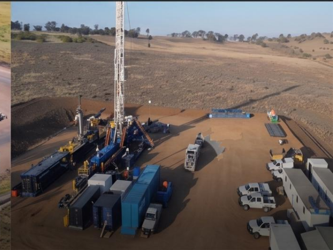
Siruction Well Drilling Site
